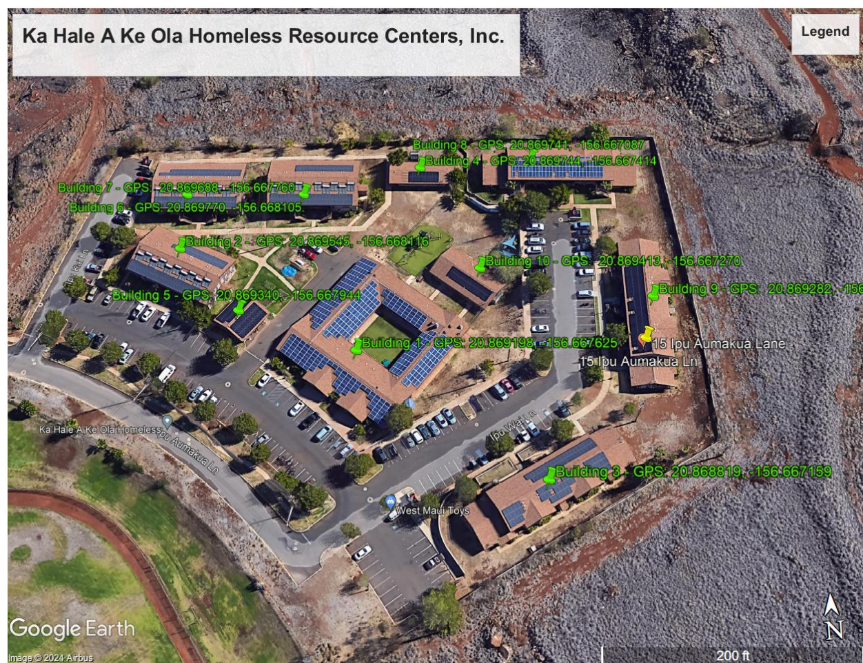
Figure 1: KHAKO Westside Before Damages
