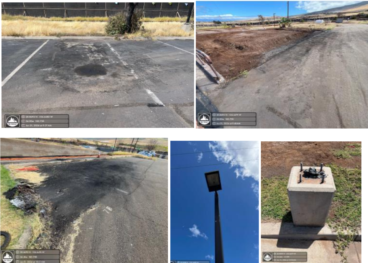
Figure 3: Parking Lot Damage
